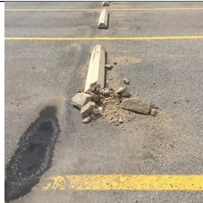
P9. Crossland: Broken bus parking back stops
